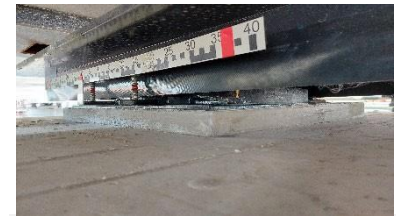
Conbextra BB installed below Viaduct bearing plate
