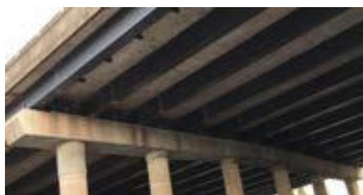
Oldbury Viaduct, M5 Midlands
