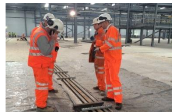
Site visit carried out to assist with smooth installation
