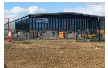
Exterior of factory
