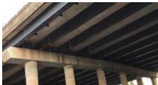
Oldbury Viaduct, M5 Midlands
