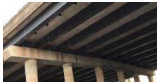
Oldbury Viaduct, M5 Midlands
