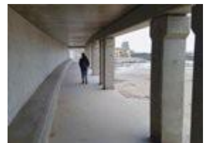
Finished base & precast columns
