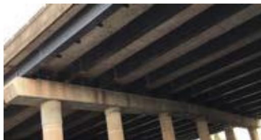
Oldbury Viaduct, M5 Midlands
