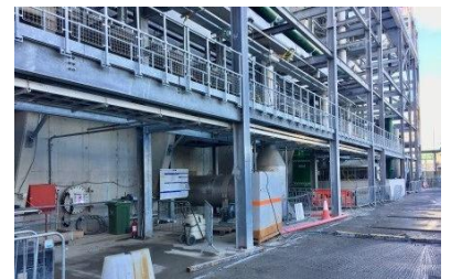
Mechanical and pipework installation
