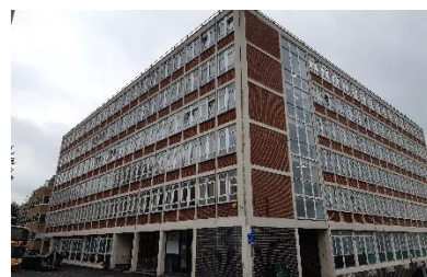
Before – front elevation of building
