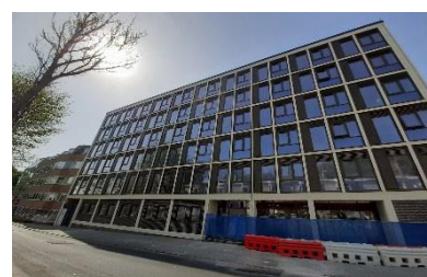
After: the finished result with improved exterior finish
