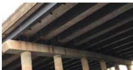
Oldbury Viaduct, M5 Midlands
